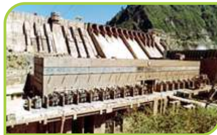
On 5th April 2012. 6th Sem students visited Salal Hydel Power Station
